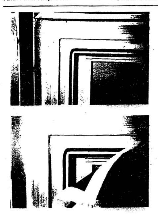
Photographs #1 & #2 - Velcro hook and felt system with closed cell rubber gasket.
